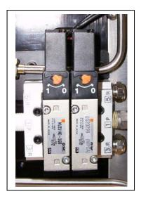
Figure 1 – The previous Reamer Solenoid Valve is shown in figure 1a (to the left) and the NEW Reamer Solenoid Valve (also SMC brand) is shown in figure 1b (to the right). The NEW product is rated IP65 for improved protection from harmful welding environments.
