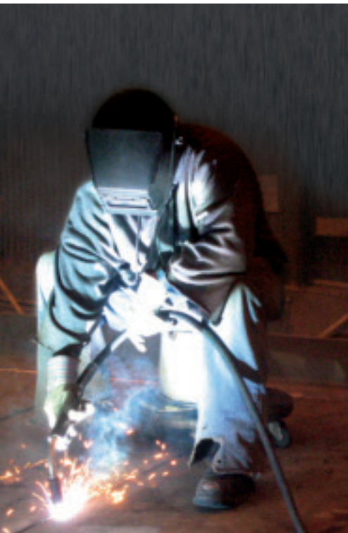
Fig. 1 — A welder is shown using the gas metal arc process. Selecting the proper shape, style, and material of nozzle for a given welding application can help minimize downtime, reduce costs, and improve weld quality and productivity.
